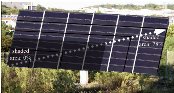
Fig. 20. PV-array with 6 strings of 9 CIS modules each one(UTM 29T 525820.68E 466832.28N).
